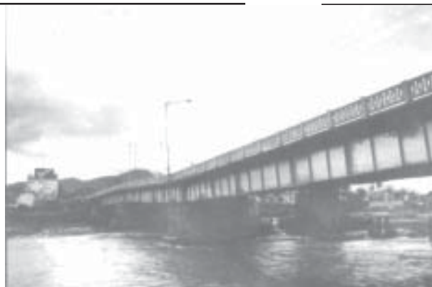
After collapsed Pier
